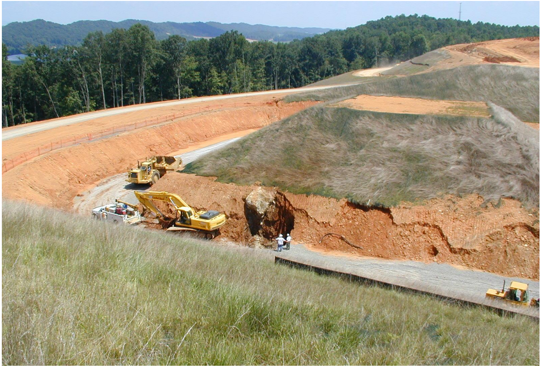
Collapse in excavation for SNS (Spallation Neutron Source) ring
